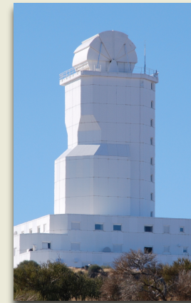
Vacuum Tower Solar Telescope Tenerife 0.7 m 10 cm subap. 37 act. 2.1 kHz
